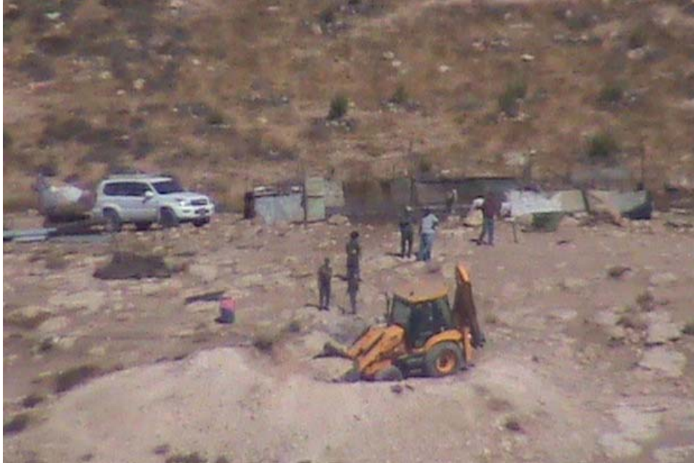
Israeli bulldozers demolish water cistern in Zenuta August 28, 2012 (Operation Dove)
