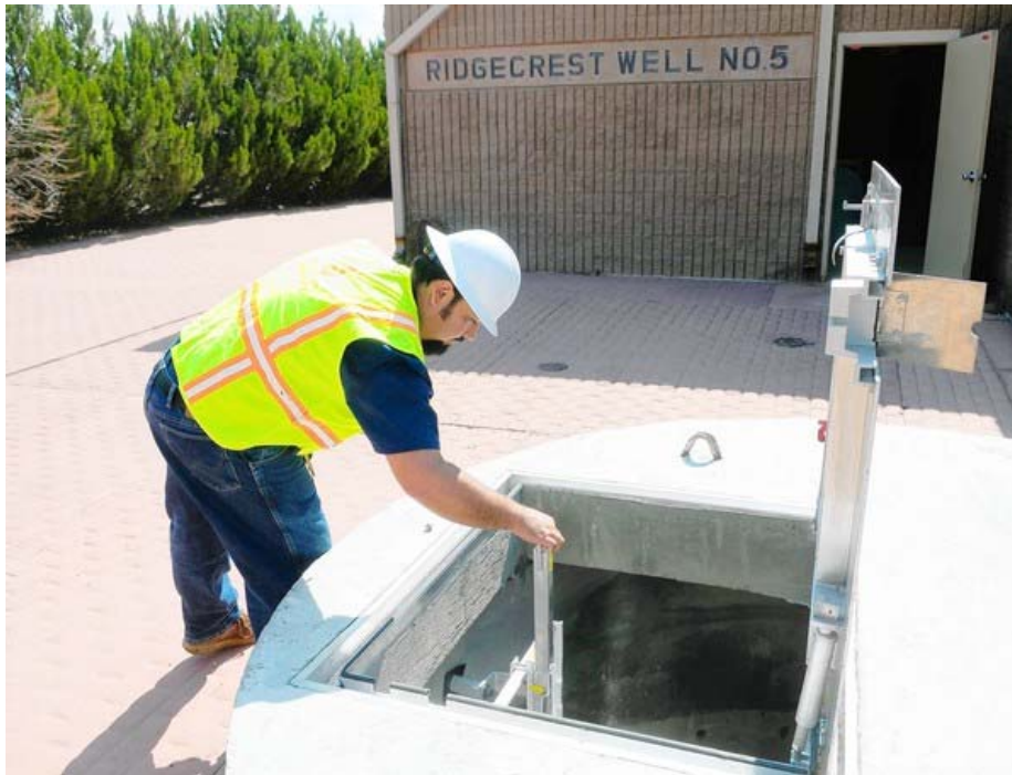
Technician James Baca performs maintenance work at an Albuquerque well near the leak site at Kirtland Air Force Base. (Adolphe Pierre-Louis, Albuquerque Journal / July 11, 2012)
