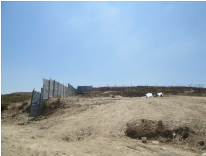
Water project work site (Photo by IWPS)
