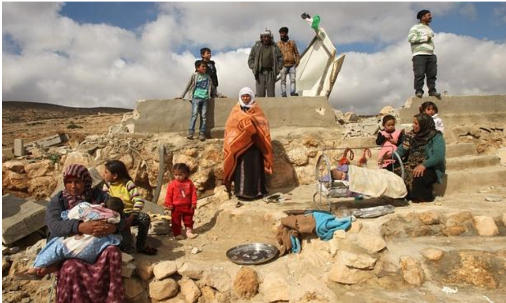
A distraught Palestinian family amid the remains of their home after it was demolished by Israelis in Musafir Jenbah. Photograph: Hazem Bader/AFP/Getty Images
