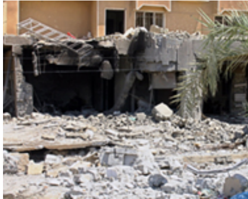
Some 13 houses were destroyed
