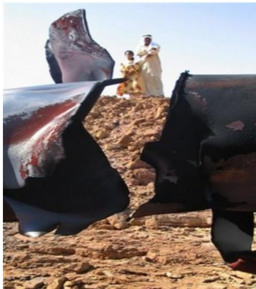
Pipeline outside Baji, near Tikrit, Sept. 5, 2005. Insurgents detonated a gas pipeline connecting Ujil field with Baji refinery. (AP Photo/Bassim Daham)
