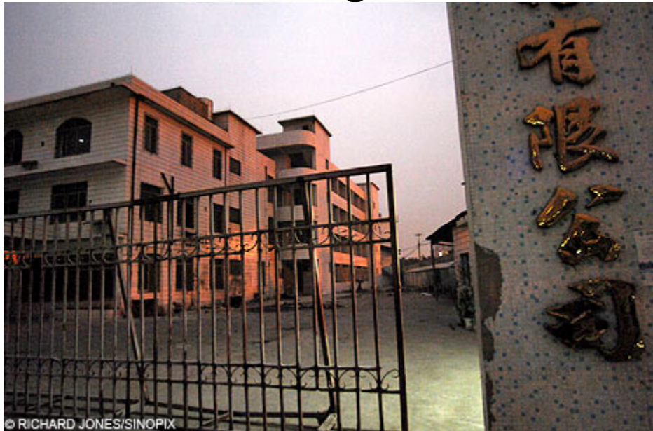
The wrecked Dingfu factory after it was destroyed by the workers.
