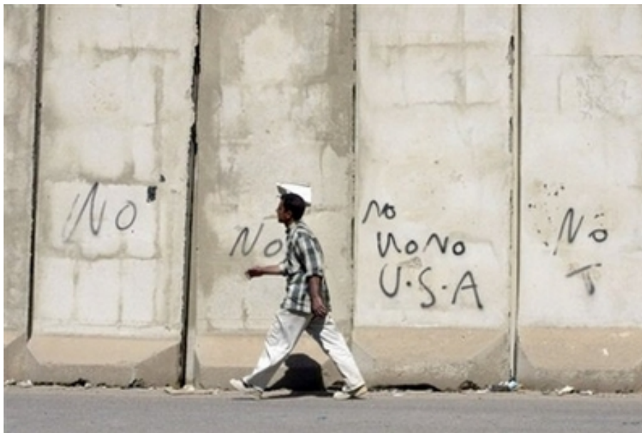
A concrete block wall surrounding a neighborhood in Baghdad in March 2008. (AFP/File/Ahmad al-Rubaye)
