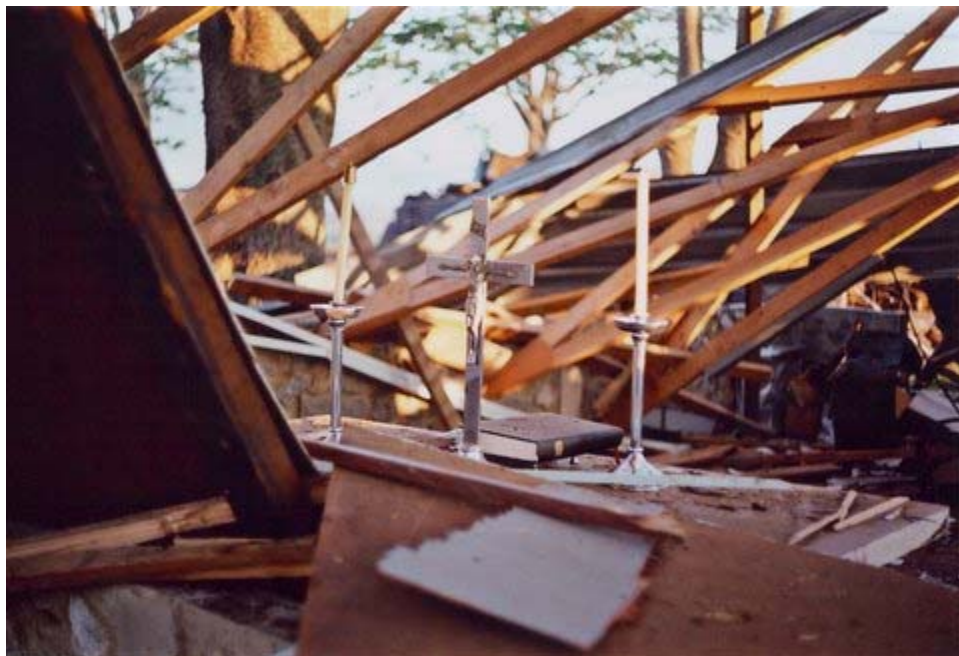
Small A-frame chapel destroyed by explosions--An Khe, Vietnam April 1971
