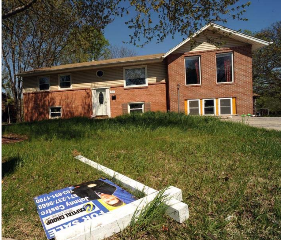
Squatters were removed from this vacant home located on West Maple Ave. in Sterling. (Photo: Tracy A. Woodward)
