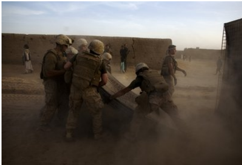
March 15, 2010: In Marjah, marines of the First Battalion, Sixth Marine Regiment build a barrier around their base. (AP Photo/Dusan Vranic)
