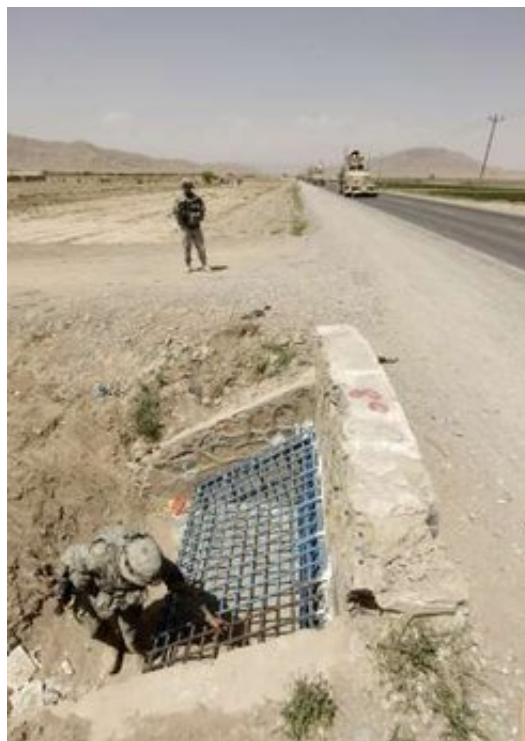
Soldiers from the U.S. Army's 20th Battalion, 584 Mobile Augmentation Company (MAC), Route Clearance Patrol (RCP) inspect a security grill fitted over the end of a culvert in Kandahar April 2, 2010. The security grills assist in preventing the placement of improvised explosive devices (IEDs) in drainage culverts. REUTERS/Tim Wimborne
