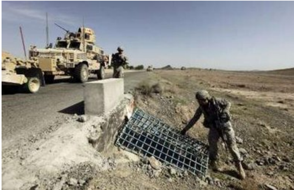
Soldiers from the U.S. Army's 20th Battalion, 584 Mobile Augmentation Company (MAC), Route Clearance Patrol (RCP) inspect a security grill fitted over the end of a culvert in Kandahar April 2, 2010. The security grills are supposed to assist in preventing the placement of IEDs in drainage culverts. Reuters/Tim Wimborne
