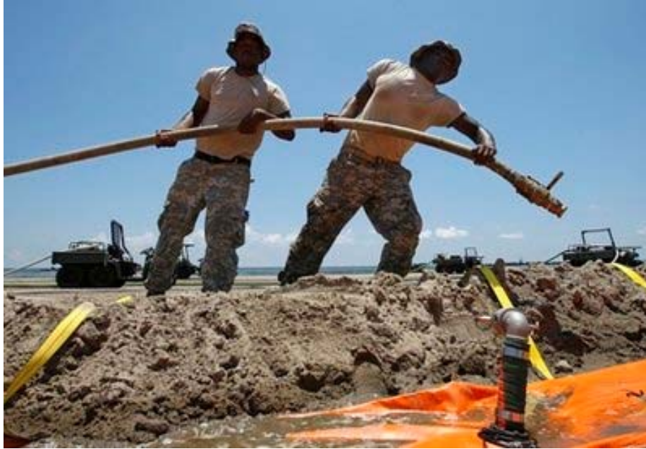
Louisiana National Guard Specialists Alvin Dunn and Bryan Jones carry a hose to fill a tiger dam on a beach in Grand Isle, La., June 1, 2010. When completed, the water-inflated dam is expected to protect the island's entire shoreline along the Gulf of Mexico. (AP Photo/Patrick Semansky)
