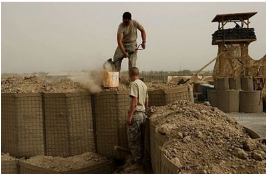
Jul 27: US soldiers fill a barrier as they build a watch tower at a forward operating base in Dand district of Kandahar Province in Afghanistan. (AFP/Manpreet Romana)
